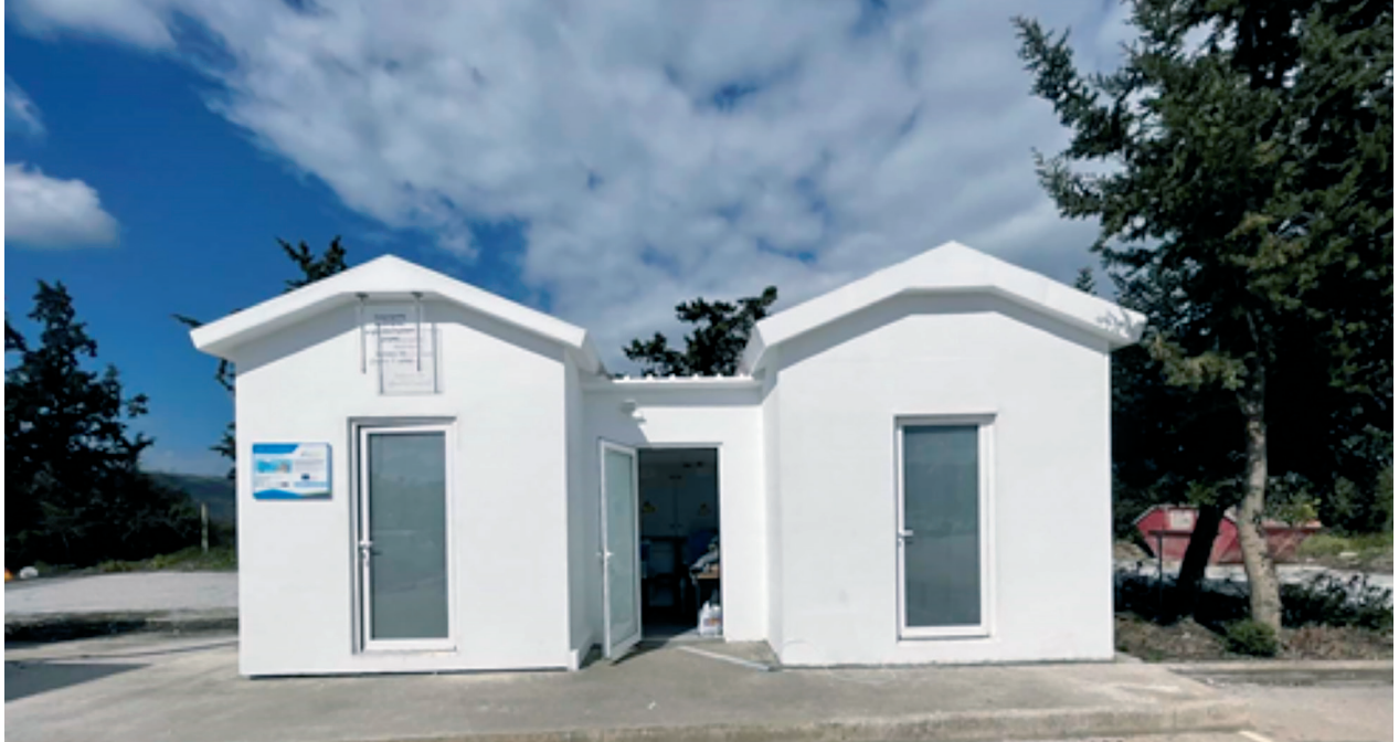
Figure 11 The Demo House in Crete
